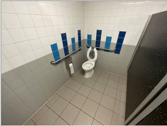
TOILET STALL OVERVIEW
