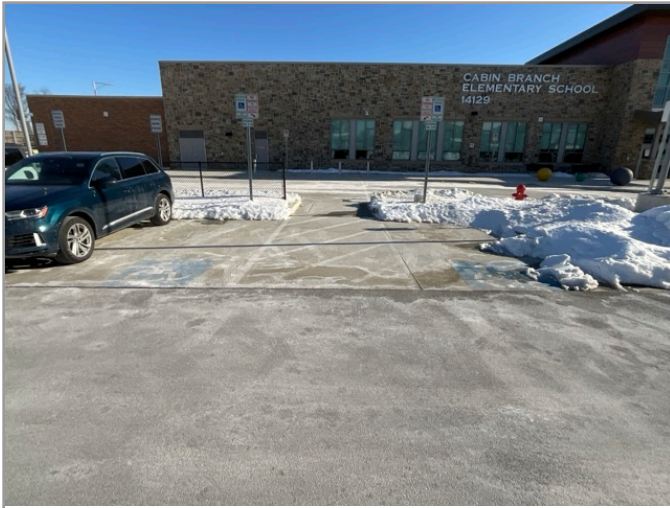
OVERVIEW OF ACCESSIBLE PARKING AREA
