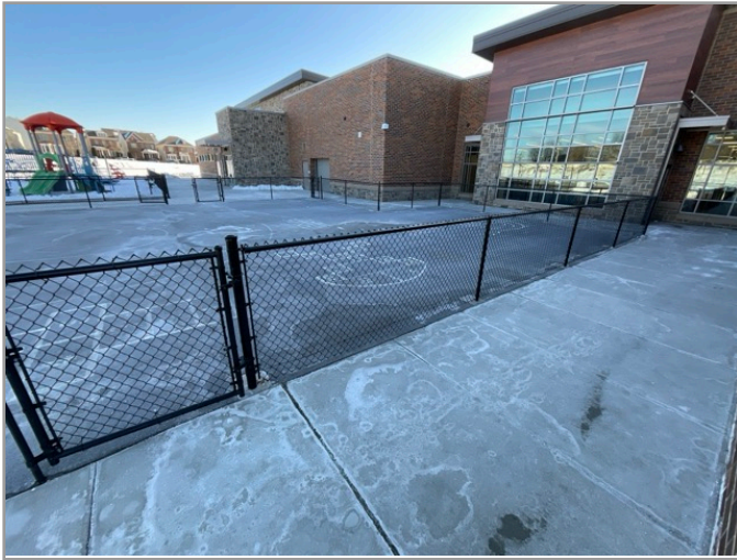
ACCESSIBLE ROUTE TO PLAYGROUND
