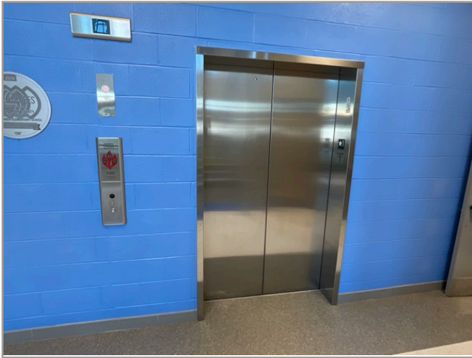
LOBBY LOOKING AT CABS
